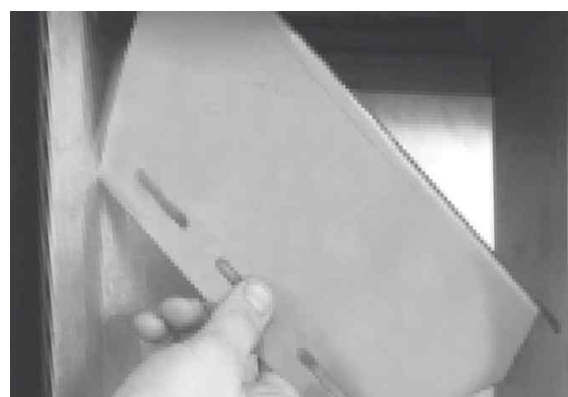
Figure 14. Remove the fire protection plate
